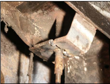
Figure 3: Typical Front Mounting Cracked in Half
