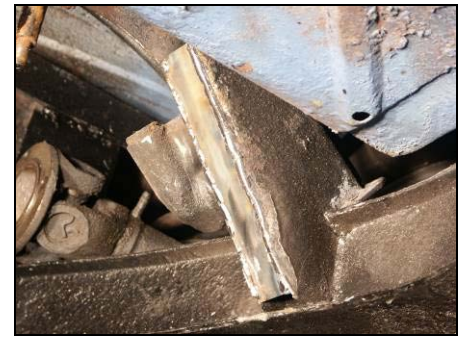
Figure 17: Item 2 Welded in Place to the Rear Bridge Body Fitted
