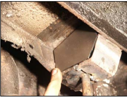
Figure 12: Item 3 Placed on the Forward Bridge Body Fitted
